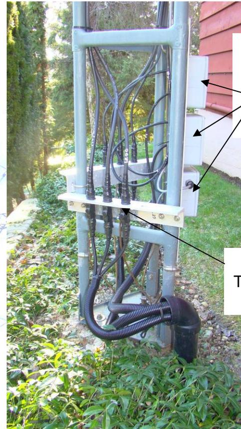
150 V Gas Tube Wire Suppressor Enclosures
